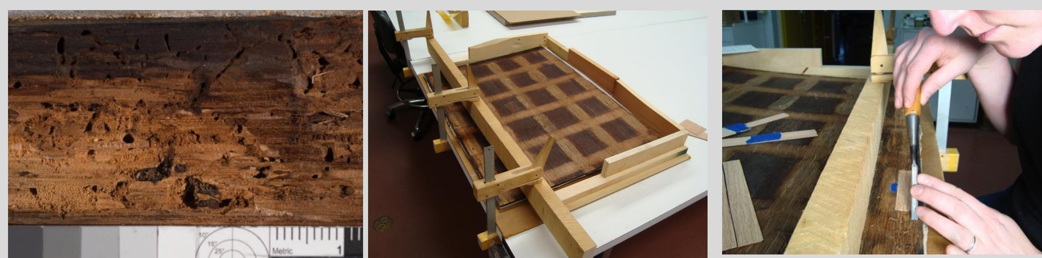
Detail of insect damaged wood
